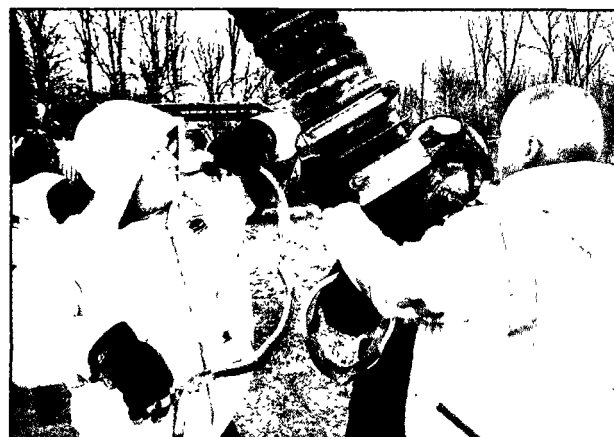
Canton DPW staffers Curt Foster and Dave Arnold clamp the hose on the Vactor truck.
