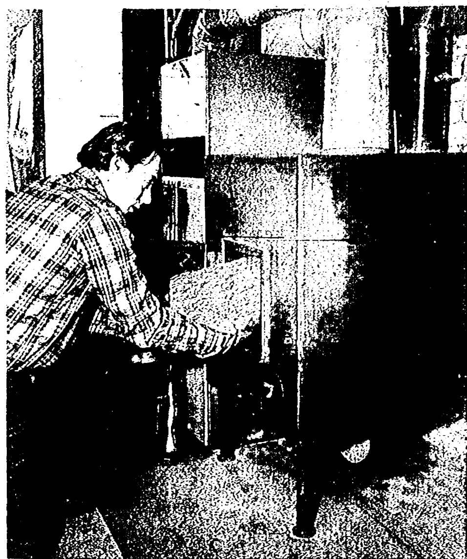
Mike Mangan loads up the stove he built at his Garden City home that uses his furnace blower system to circulate the heat.
